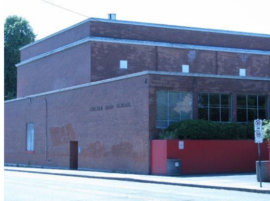
Gymnasium (120A), looking southeast.
