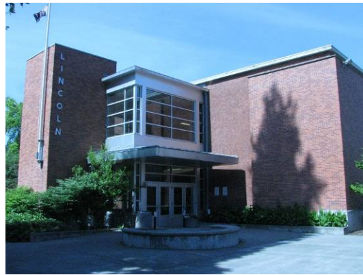
New entrance on west side of building (120A).
