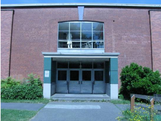
East elevation (rear) entrance (120A).
