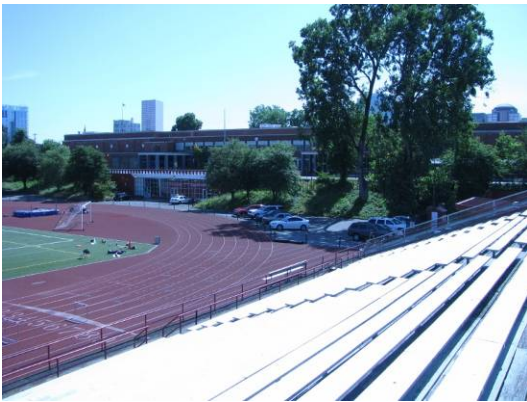
West elevation (120A), looking east.
